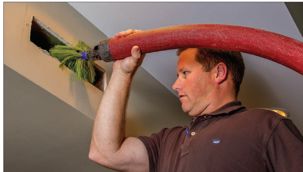
DUCTS MAY need to be serviced by professionals in homes where indoor air quality is poor.
