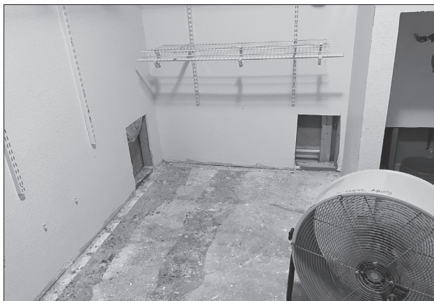
SERVPRO USED special fans to dry out the room.
